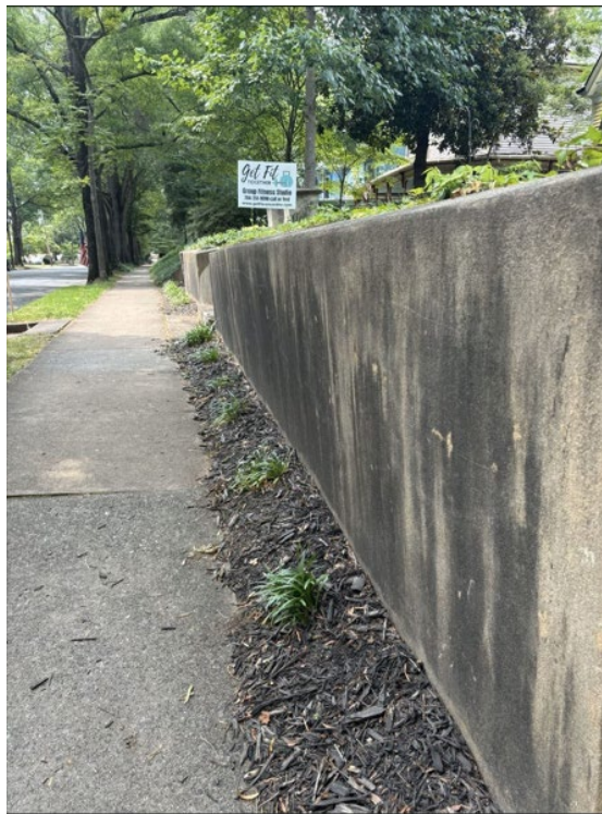
Wall facing North (right side nearest)
