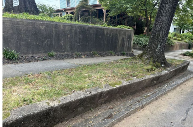
Right side wall
