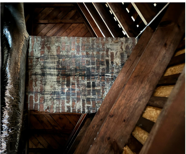
View in attic
