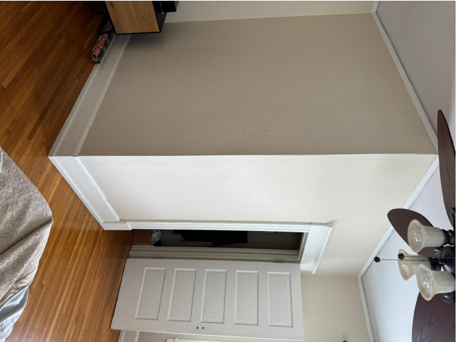
2nd floor closet with chimney inside
