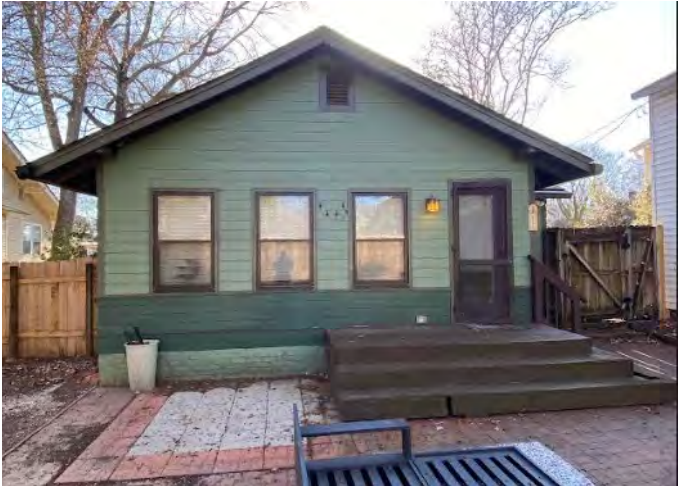
Existing rear of home:
