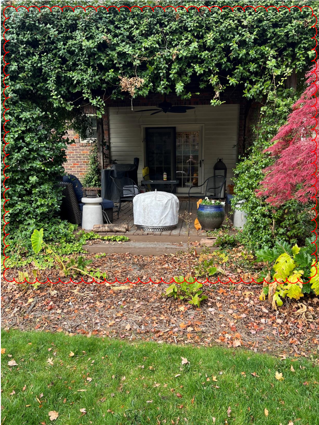
Existing Deck and Pergola to be Removed
