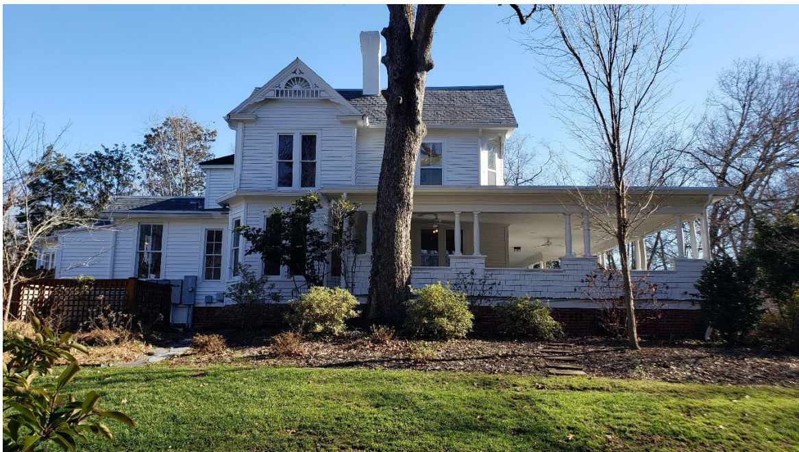
Existing House: View from Left Side
