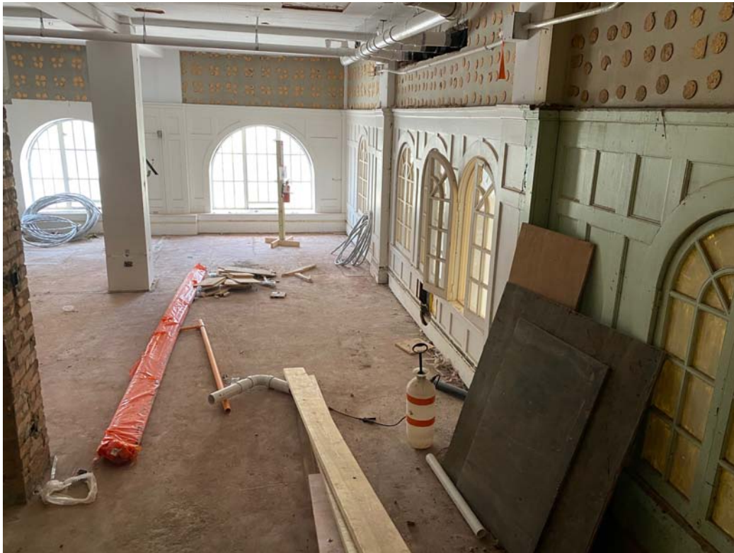
Tenant space interior - rear mezzanine (57 Union Street S.)
