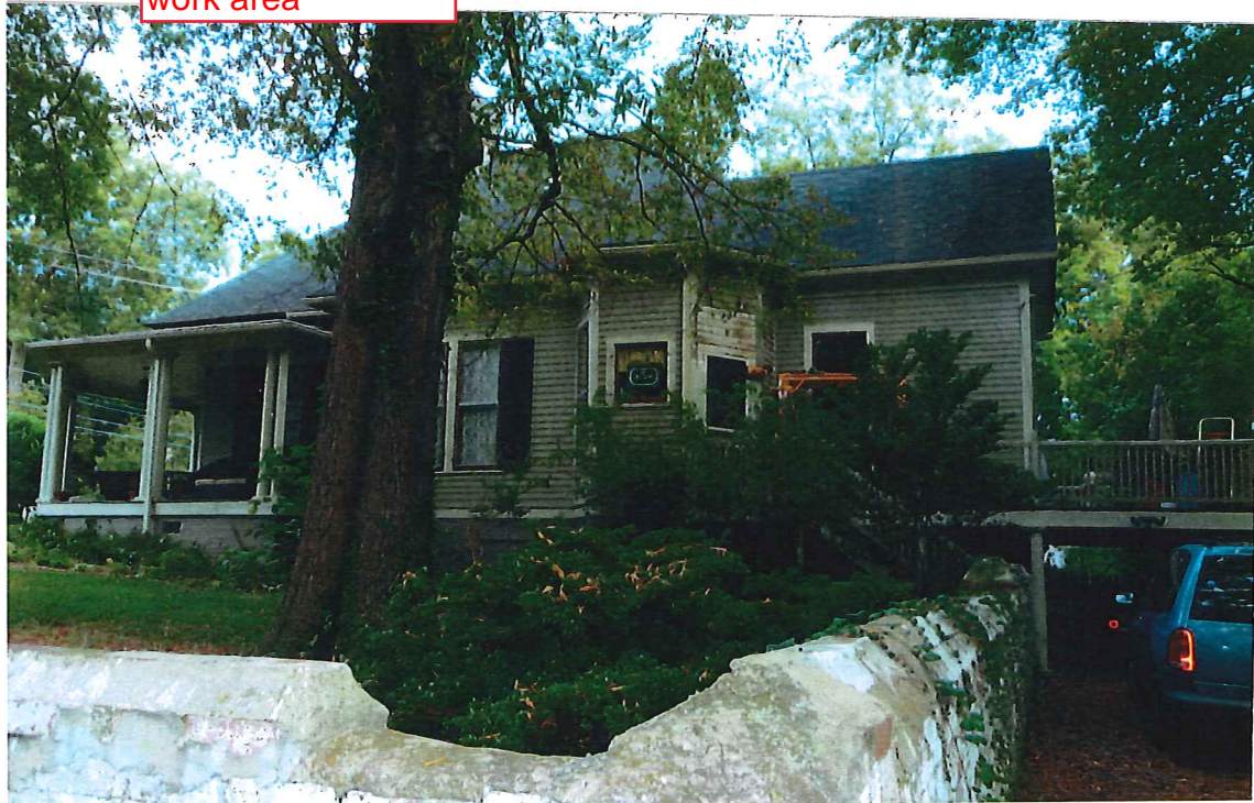
Franklin Street-- work area
