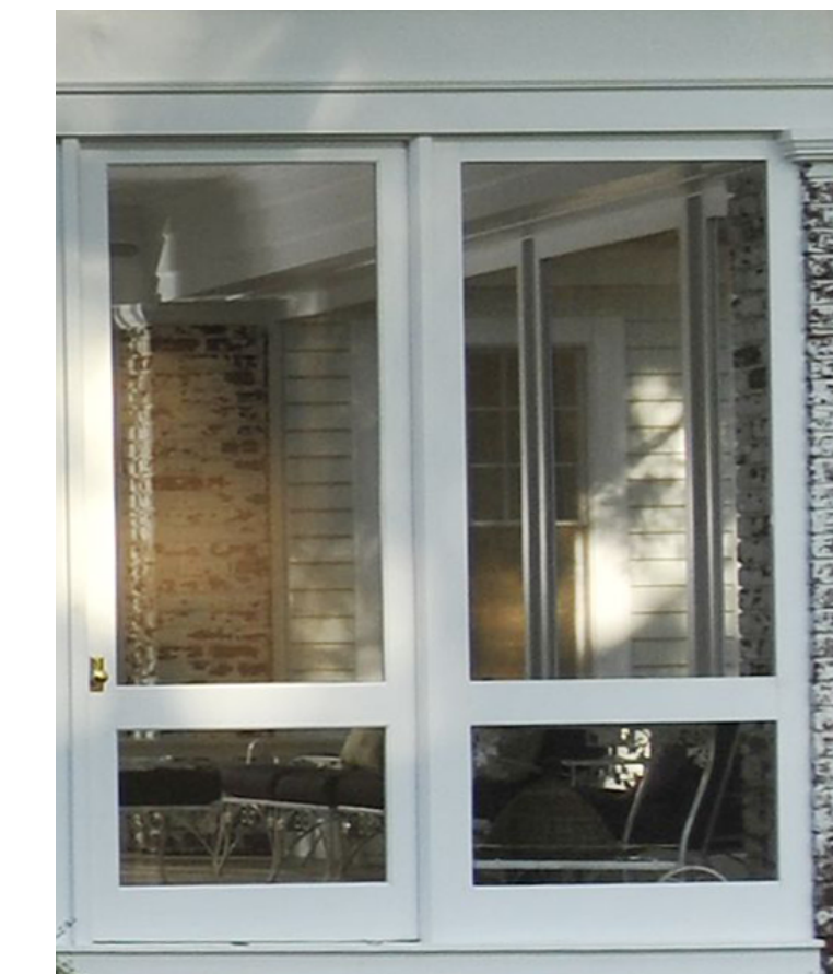
Fiberglass Screening Within Cedar Wood Sash (New Screen Porch Addition)
