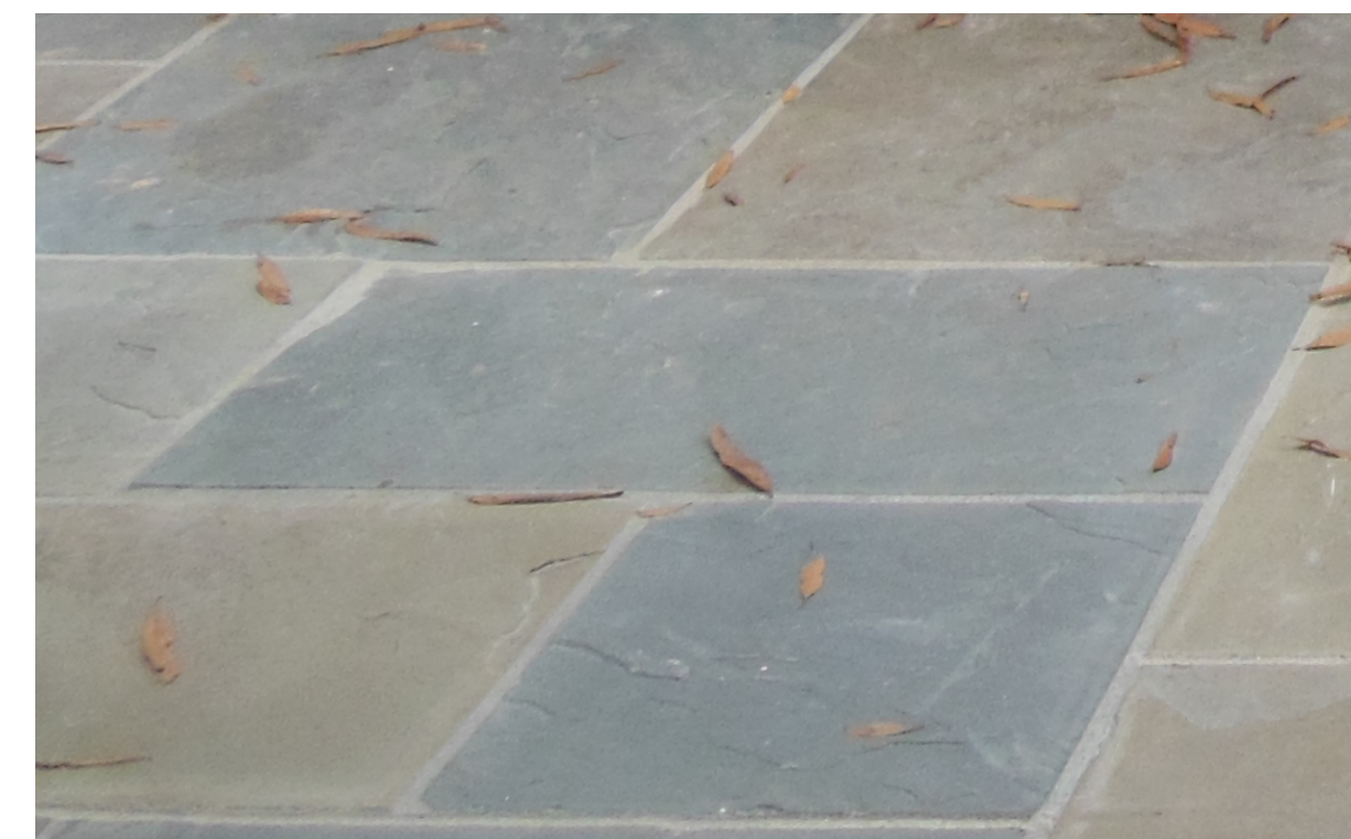
Bluestone Paver (Ashlar Pattern; New Covered Porch, Raised Terrace & Patio)
