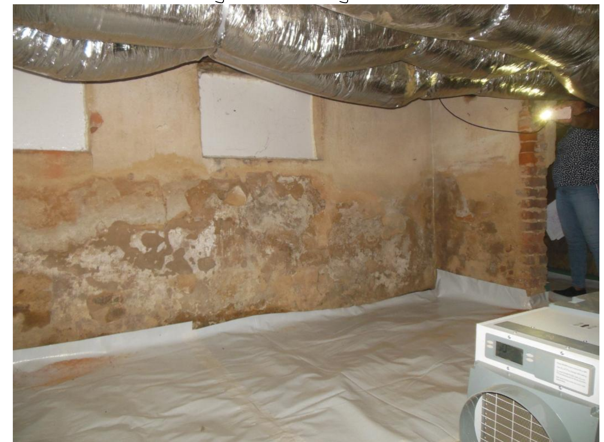
Rear Suite House Basement (Existing - 'Before')
