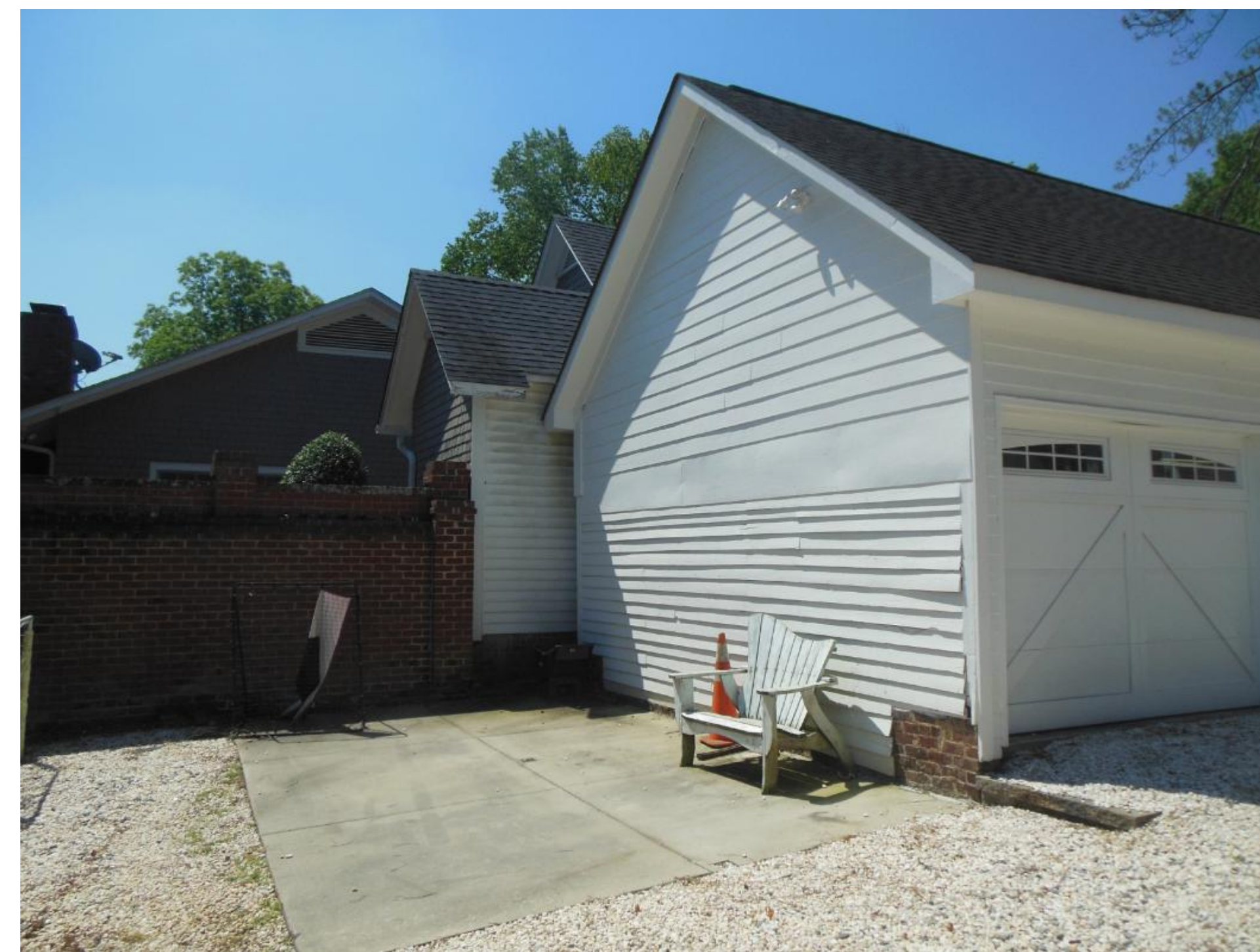
Rear Garage Elevation (Existing - 'Before')
