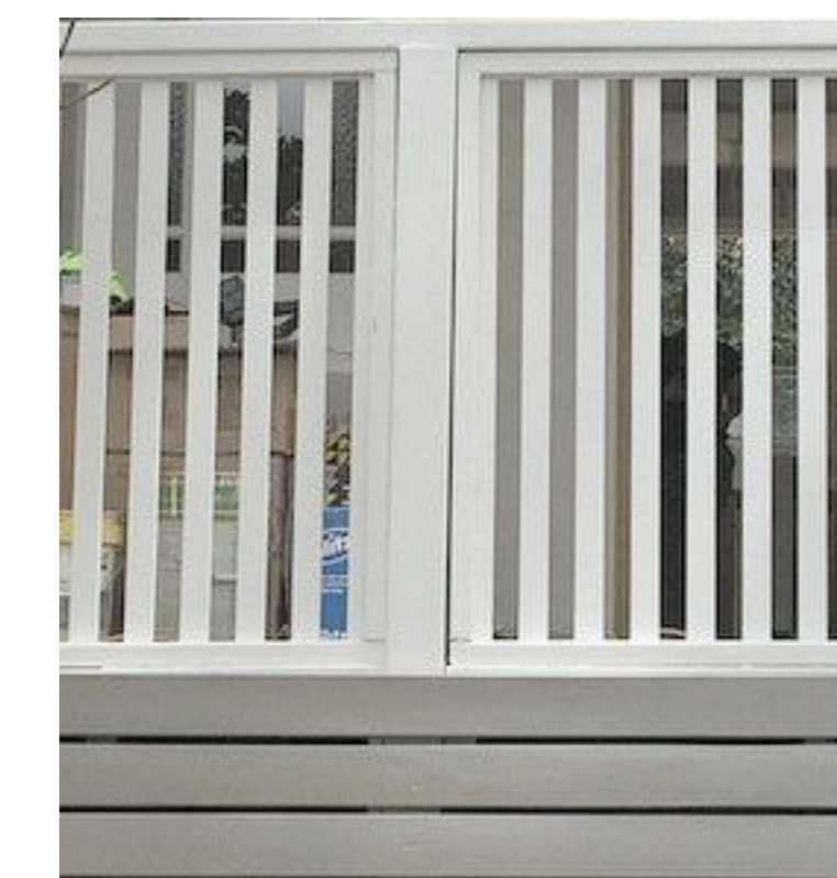
P.T. Wood Railing & Screening (New Exterior Stair/Landings; Rear of Garage)
