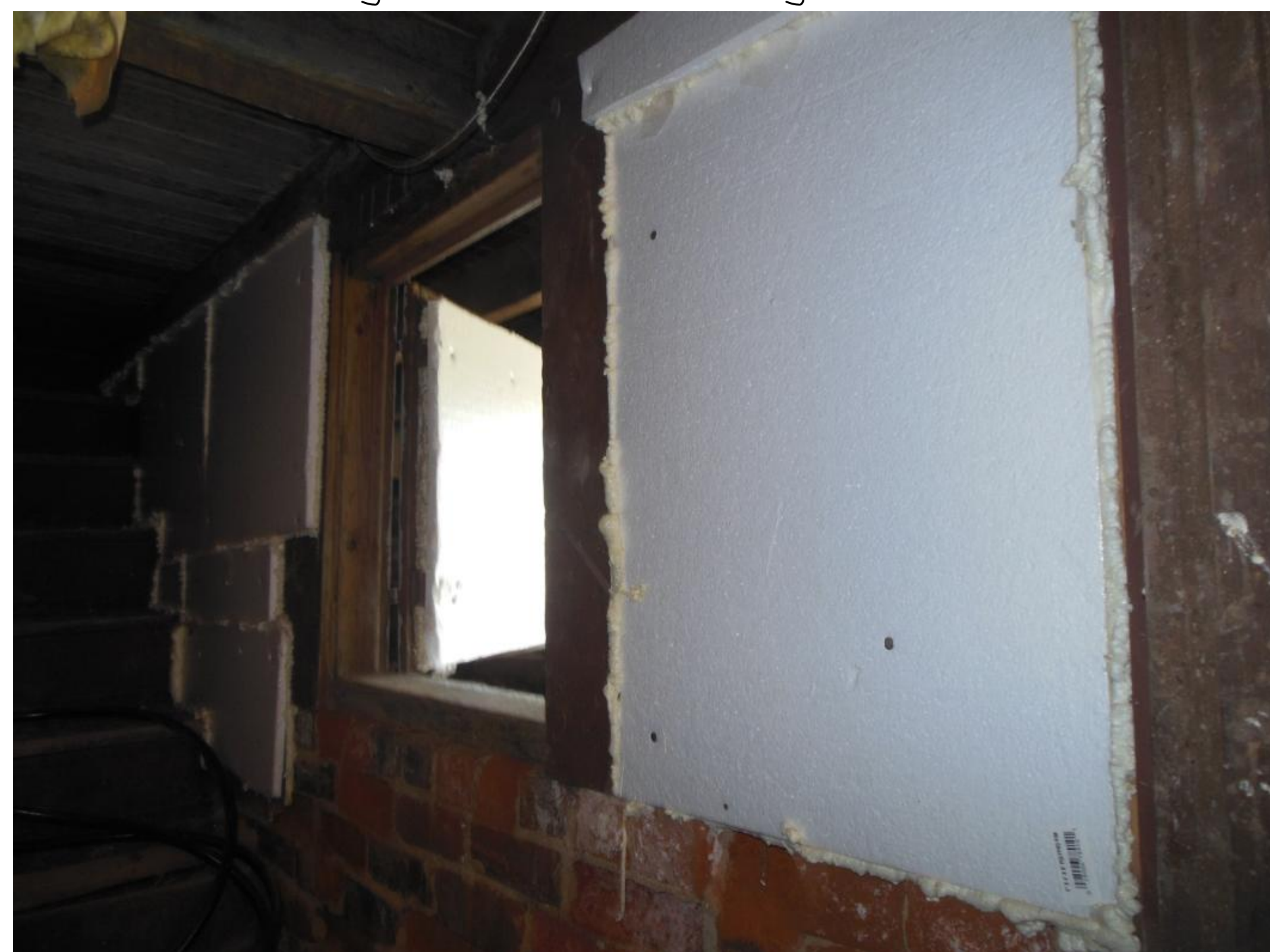
Rear Suite House Basement Access (Existing - 'Before')
