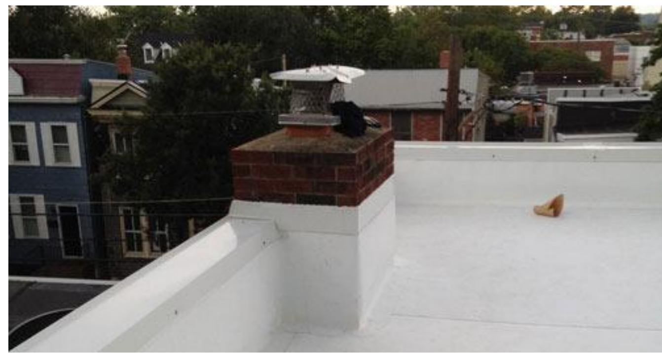
TPO Roof Membrane Equal to Firestone - UltraPly (New Porch Low-Pitch Roof; White Finish)
