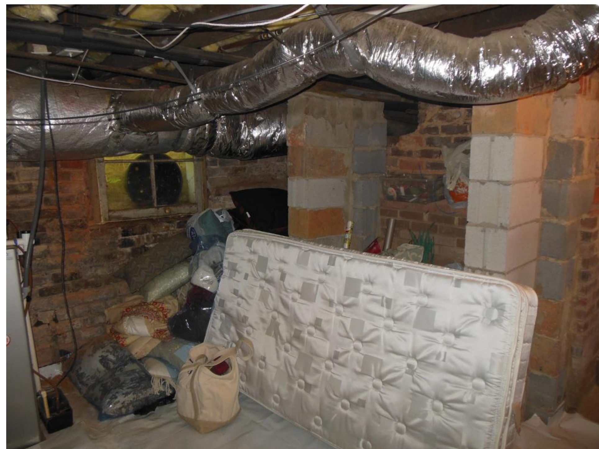
Original House Basement (Existing - 'Before')
