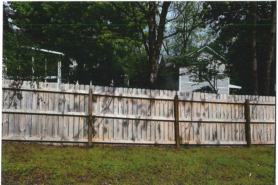
Existing west side fence
