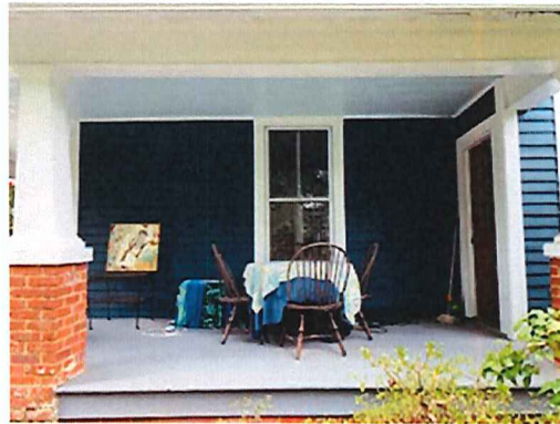
Side view – area will be enclosed – with windows That match look of window shown
